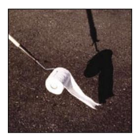
Some cracksealing work is blotted with tissue paper, applied with a rolling tool.
