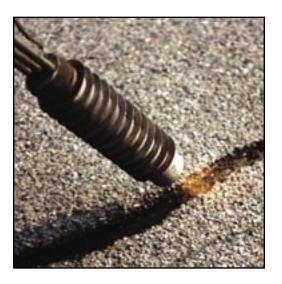
A hot air lance, or heat lance, combines super heated air with compressed air to clean the crack sides, remove moisture and heat crack sides to create a better surface for sealant adhesion.
