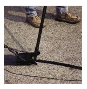
Sealant should never set higher than 1/8" above the pavement level. V-shaped squeegees allow crews to flatten the sealant over the crack and remove excess. This is a particularly important step when cracksealing pavement that will eventually be overlayed with SuperPave.
